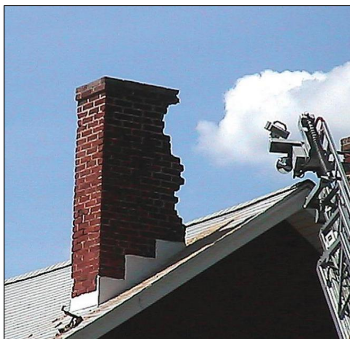
Figure 3.1.6.3.1: Chimney Damage (Fayetteville, PA) - Aug 2011 Earthquake 54
