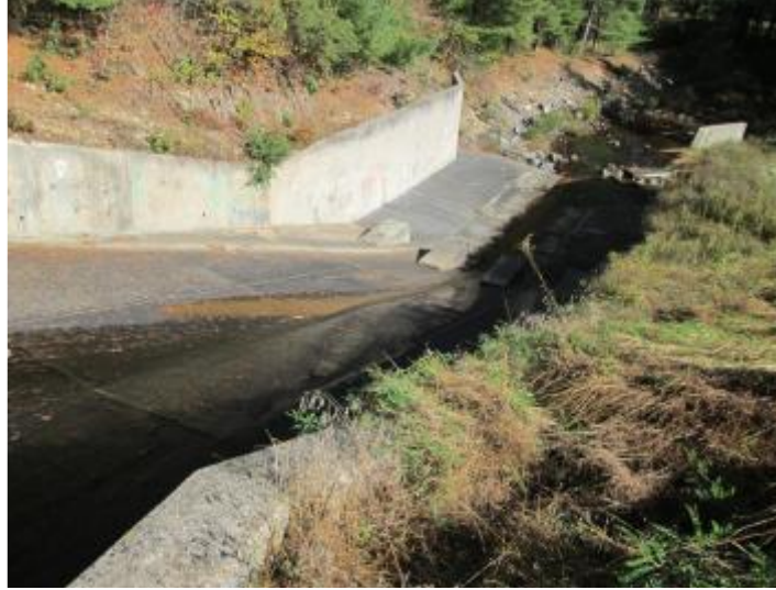
Figure 3.1.4.5.17: Carbaugh Run Dam Spillway
